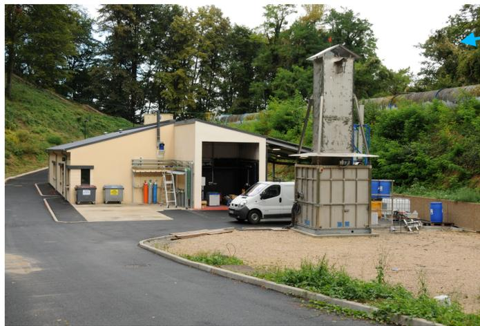
240 m<sup>2</sup> of new laboratories dedicated to battery safety, with secured test chambers (admissible overpressure : 1 bar) and environment protection equipment in relation with pollutant releases during test (gas cleaning unit)
