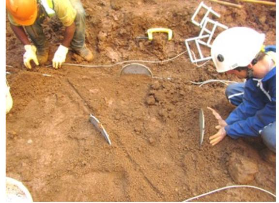
**O**ur services are based on strain gauges, total pressure cells, pore pressure sensors, flat jack cells, clinometers, extensometers and any combination of these sensors.
